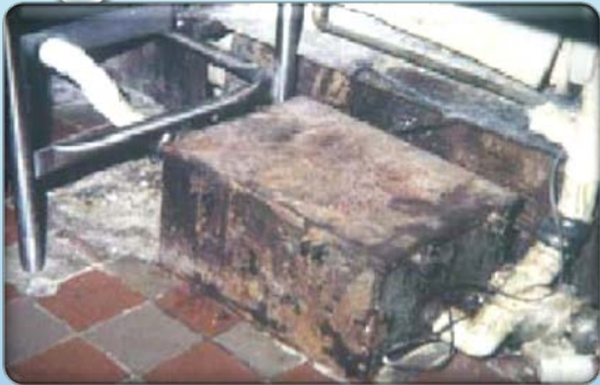
Overflowing Grease Trap
